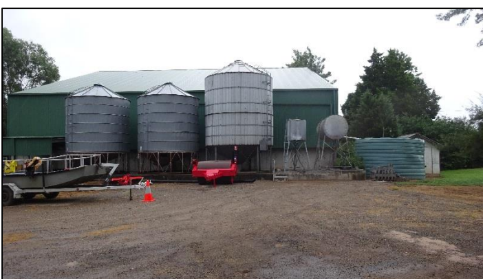
Plate 4: Two metal ASTs and three metal feed silos north of maintenance shed.
